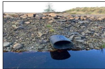
Existing track crossing looking west
