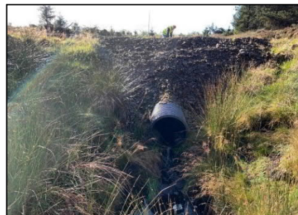
Existing crossing looking south
