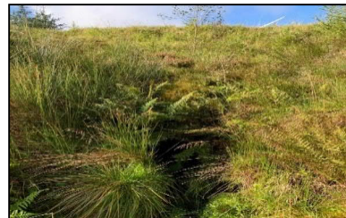
Existing crossing looking east
