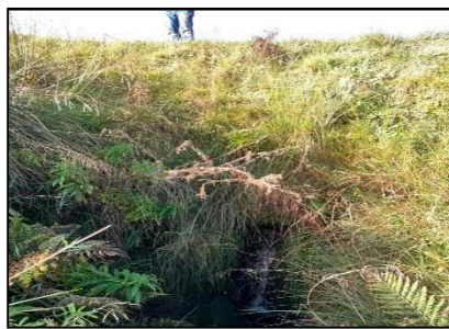
Existing crossing looking east
