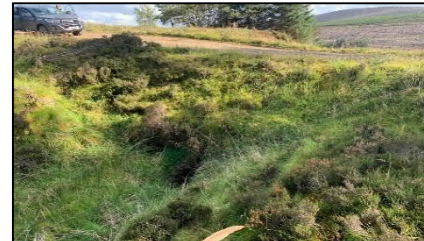
Existing crossing looking south west
