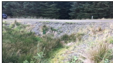
Existing crossing looking east
