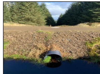
Existing crossing looking north
