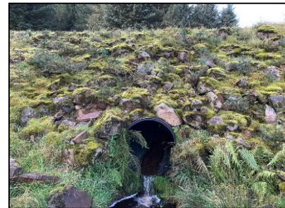
Existing crossing looking east
