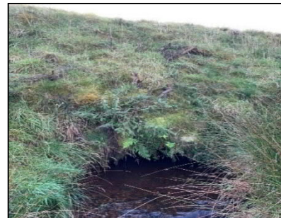
Existing crossing looking south
