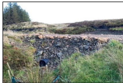
Existing crossing looking east
