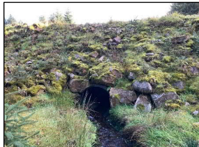
Existing crossing looking west
