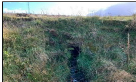
Existing crossing looking north west
