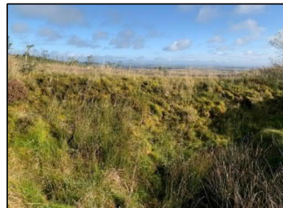
Existing crossing looking east
