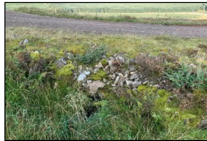
Existing crossing looking south
