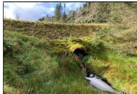
Existing crossing looking south west
